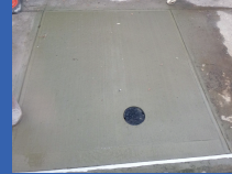
Permanent Sidewalk Repair
