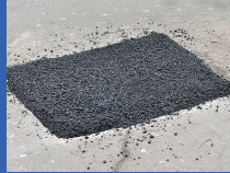
Temporary Asphalt Repair
