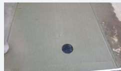
Permanent sidewalk repair at the curb stop.
