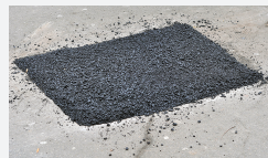
Temporary asphalt repair patch in street and/or sidewalk after service line replacement.
