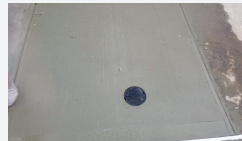
Permanent sidewalk repair at the curb stop.
